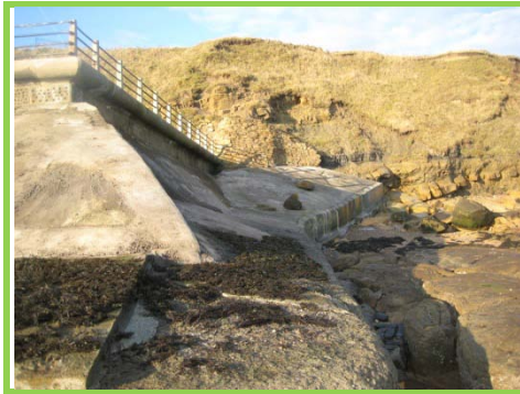
Recently repaired concrete apron at Lower Promenade seawall.
