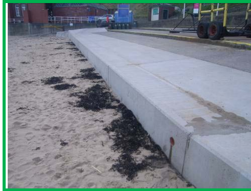
New low concrete wall along toe of wide stepped concrete apron.
