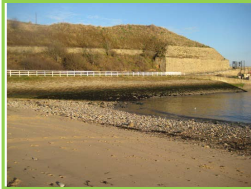
Masonry revetment at Prior's Haven in good condition
