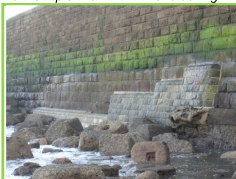
Northern pier patch repairs
