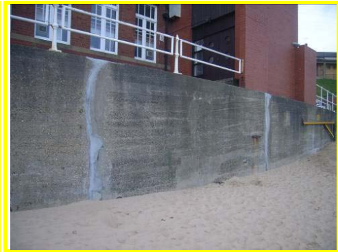
Recently repaired cracks in concrete wall in good condition.
