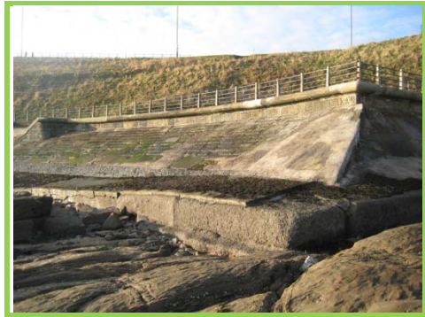
General view of northern end of wall.
