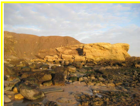
Headland cliffs at Tynemouth North Point with slumping to upper cliffs.
