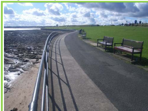
Promenade and shallow grass embankment in good condition.
