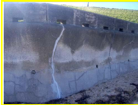
Previous repairs to crack in rendered section of seawall remain good.
