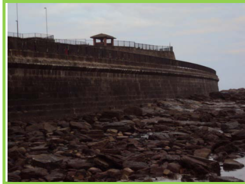
Northern wall at Browns Bay generally in good condition.
