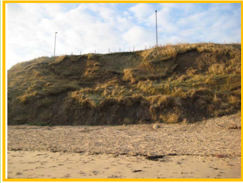
Localised slumping in need of further risk assessment.
