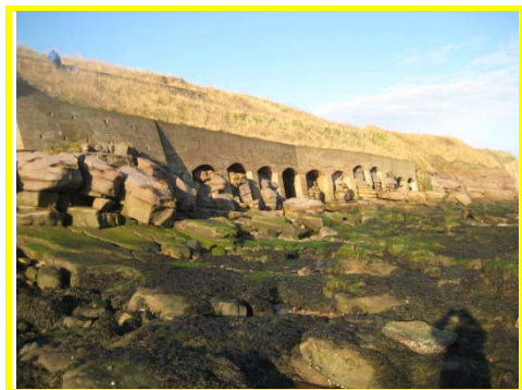
Arched retaining wall at Freestone Point
