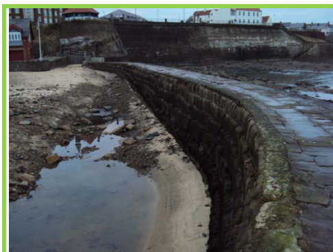
Leeward face of north pier, masonry in fair condition.
