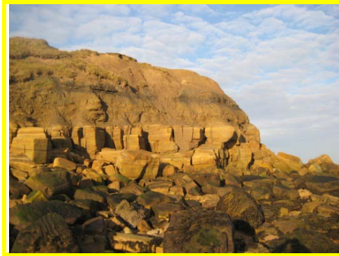
Evidence of rockfall to foreshore at Sharpness Point.
