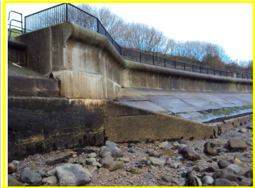
Exposed concrete toe
