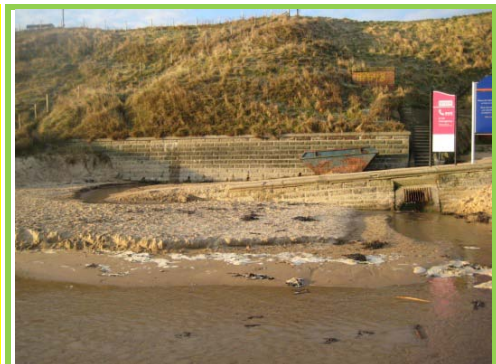
Concrete block work wall in good condition.
