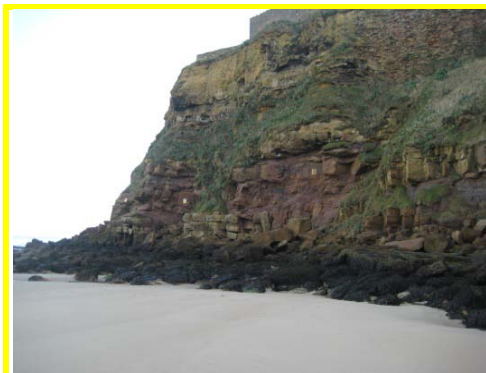
Fractured rock structure at Tynemouth Headland with rockfall on foreshore
