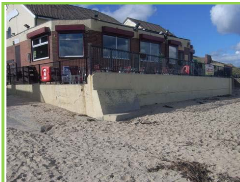
Concrete wall fronting Boardwalk Cafe in good condition.
