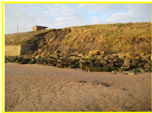
Recent slumping to southern section cliff face.
