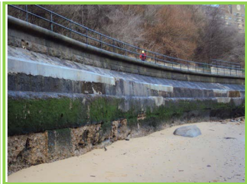
Very recent patch repairs evident throughout this section
