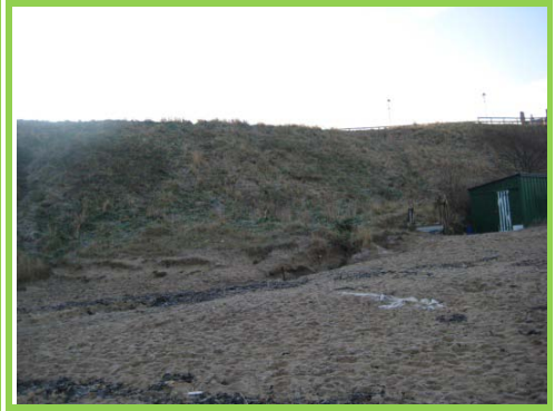
Coastal slope in good condition
