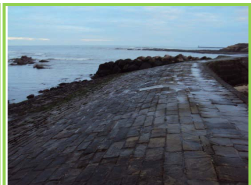
Seaward face of north pier with improved rock armour.
