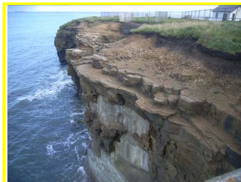
Rock falls and slippages in the overlying till at Brown's Point.
