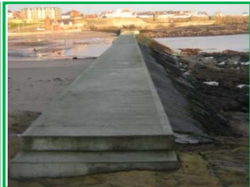
Recently repaired pier deck
