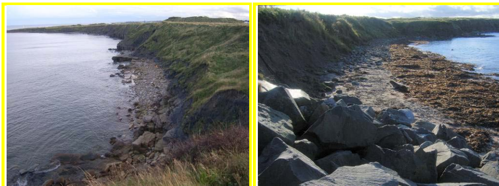
Continued rock falls and slips in cliffs north of Curry's Point.
