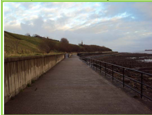
Concrete decking with occasional minor cosmetic cracks
