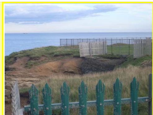
Cliff top recession to within a few meters of the boundary fence.
