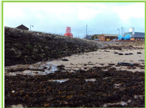
Pitched stone revetment to jetty
