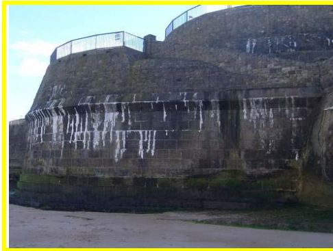
Masonry blockwork and upper masonry brickwork in fair condition.
