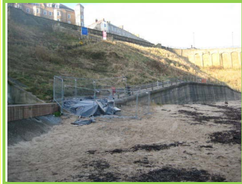
Repair works underway to access
